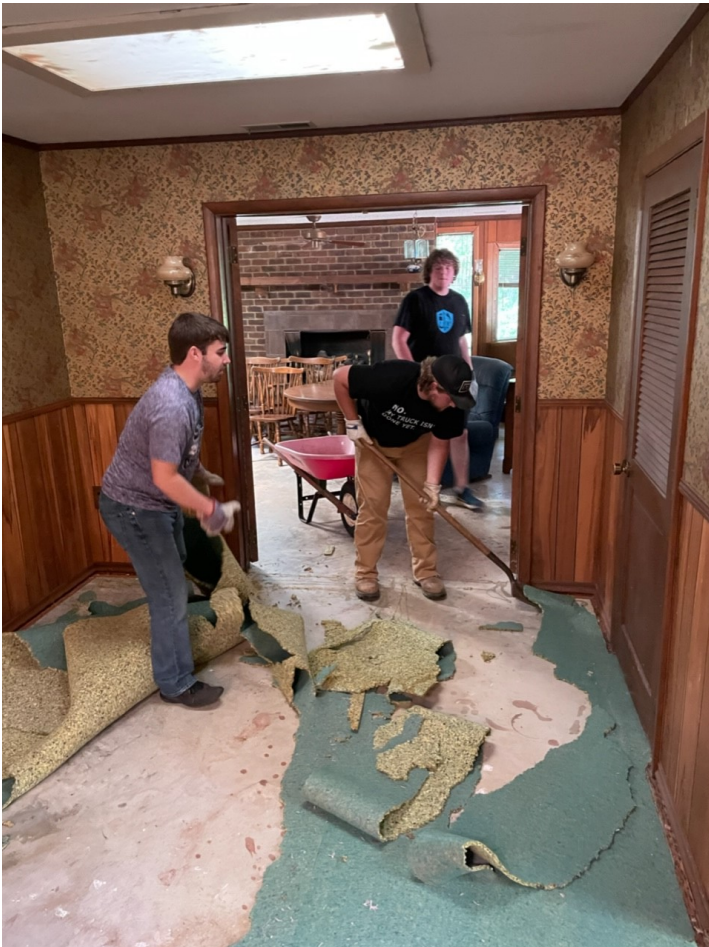
Workers renovate the UCSC facility
